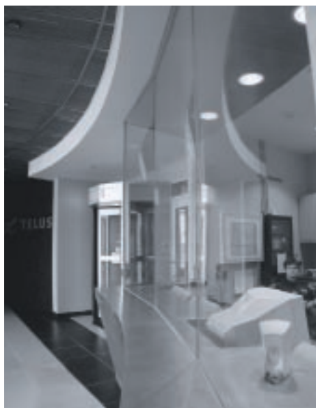
Figure 1 (left): The hardened lobby of a TELUS intelligent Internet Data Centre has bullet-resistant glass and walls, a locked mantrap, biometric scanners, and 24x7 security guards.
