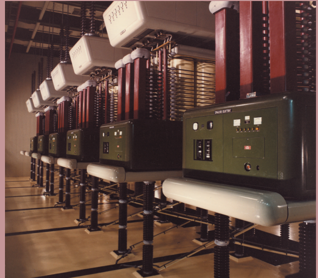
Nelson River HVDC Mercury Arc Valves
