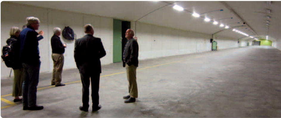
The interior hallway of one of the buildings.
