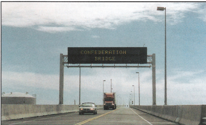
A view on the Confederation Bridge
