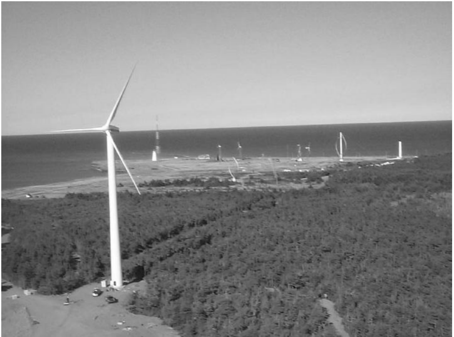
Figure 11: A view of the Windmill park in PEL. The photograph shows the 5.28 MW North Cape Wind Plant and wind test facilities of Atlantic Wind Test Site Inc. (AWTS), located at North Cape, the northernmost tip of Prince Edward Island.
