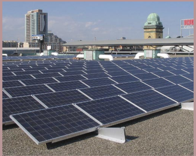
Figure 5: Exhibition Place 100KW PV system (Photo courtesy of Exhibition place).
