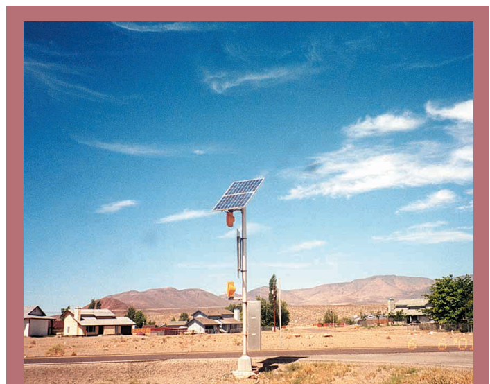
Figure 4: Small autonomous systems such as traffic signs (shown here), lights, telephones and parking meters are effective in both rural and urban areas. (Photo: Dan Ton)
