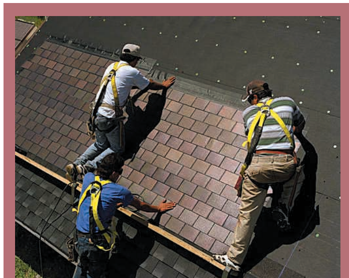
Figure 3: Photovoltaic modules in the form of shingles for roof integration. (Photo: Warren Gretz)
