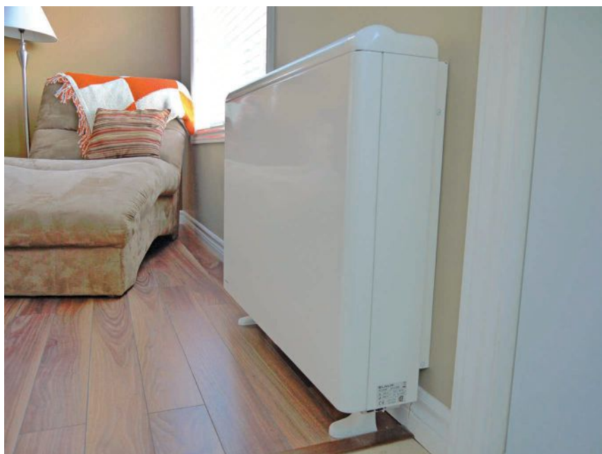
Figure 1: An Ecombi ETS unit used to replace baseboards. (Photo courtesy of Coldbrook Electric Supply; used with permission.).
