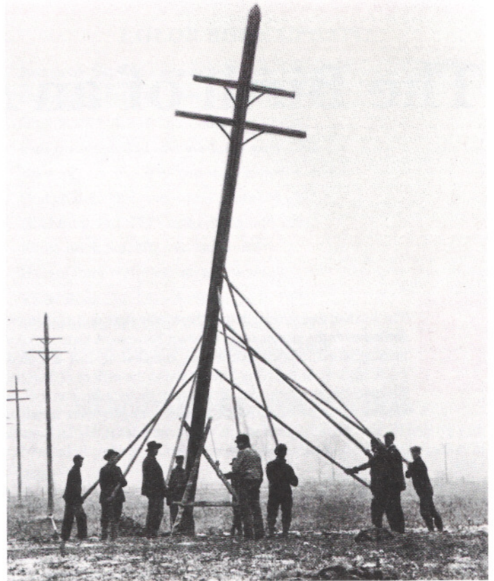
"Up she Goes" Toronto Niagara power crew erect new high voltage (12 Kv) transmission line - 1907
