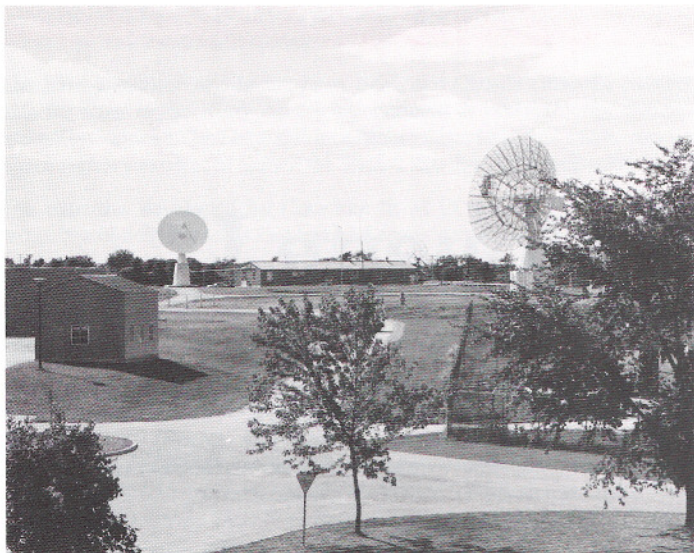
This photograph was taken in 1974 and shows the Alouette/ISIS tracking antenna (on the right), a yagi array antenna of the earlier generation and a dish antenna of later design (on the left). (Crown copyright photo reproduced with permission from the Canadian Department of Communications)
