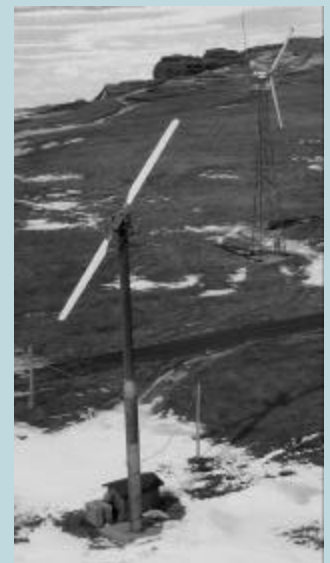
Figure 10: Lagaway LW18 80 kW wind turbine for inverter research and development.
