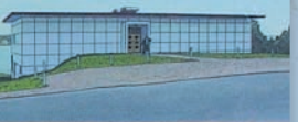
The Clarenville Cable Station, built during the Cold War, was considered a military target because it linked North America with Europe. The station had walls two feet thick to withstand enemy bombs.
