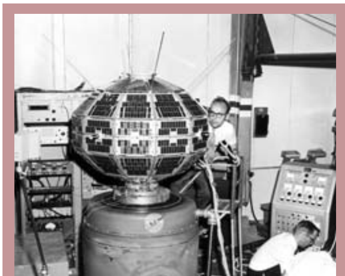
Figure 5: Alouette Vibration Testing, Goddard Space Flight Center
