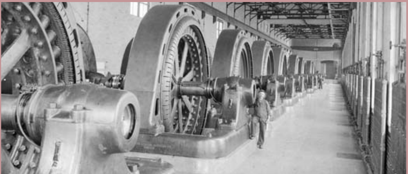
Engineering details of the Pinawa powerhouse were frugally designed: A 25-ton crane was operated by hand-chains and lighting was limited to one 100-watt incandescent bulb located beside each governor and illumination at a few other important locations.
