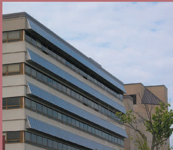
Figure 1: A 20 kW grid-connected, building-integrated PV system at Queen's University provides summer shading and year-round electricity. (Photo: Anton Driesse)
