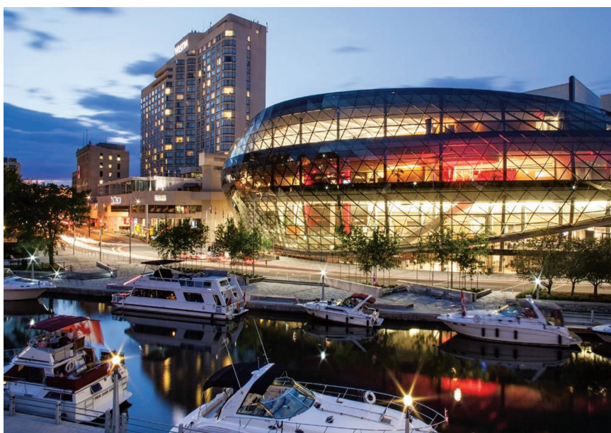
Figure 1: The Shaw Centre in the foreground with the Westin Ottawa in the background.
