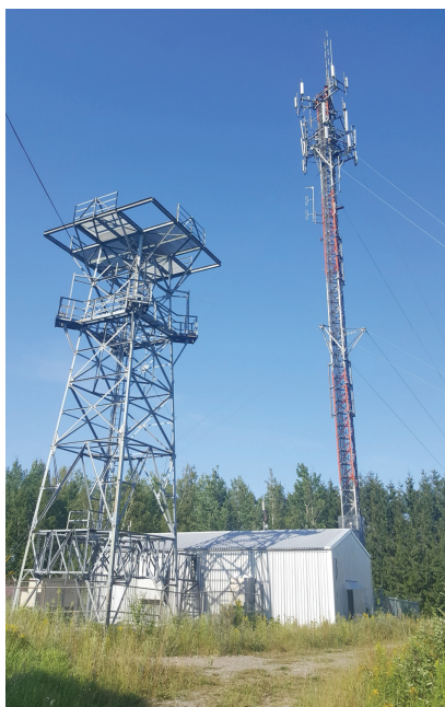
Figure 3: A recent photo of a former microwave site near Saint-André, NB, that now hosts cellular base stations.
