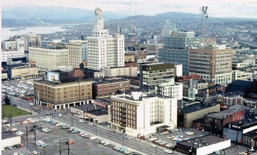
Figure 1: A 1966 photo of the Trans-Canada Microwave System tower atop the BC Tel building at the corner of Robson and Seymour in Vancouver.
